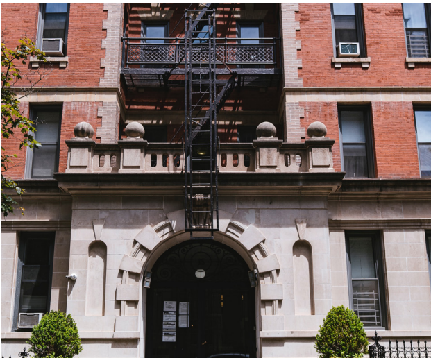
Common Entry Building
